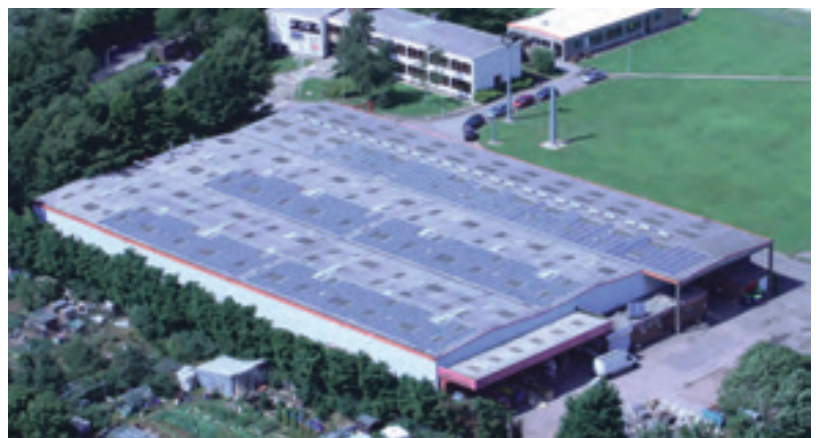
Burley's factory in Oakham with 200kW of solar panels.
