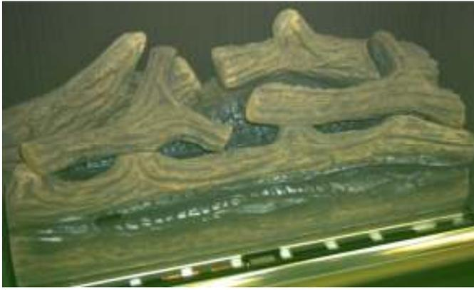
8.1.4 Place the remaining log to the right hand side of the fuel bed to bridge the front and rear log pieces. The stubby branch should nestle down and be located in the notch on the right of the rear log piece. The other end of the log shall come to rest on the branch stub
